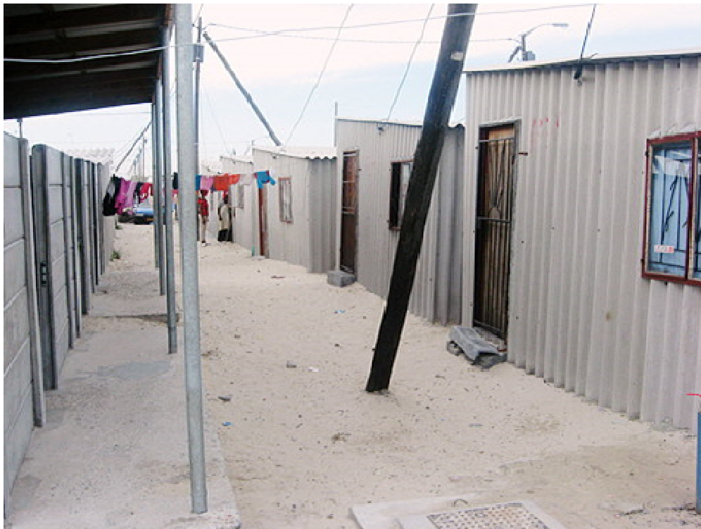
Tsunami TRA in Delft
